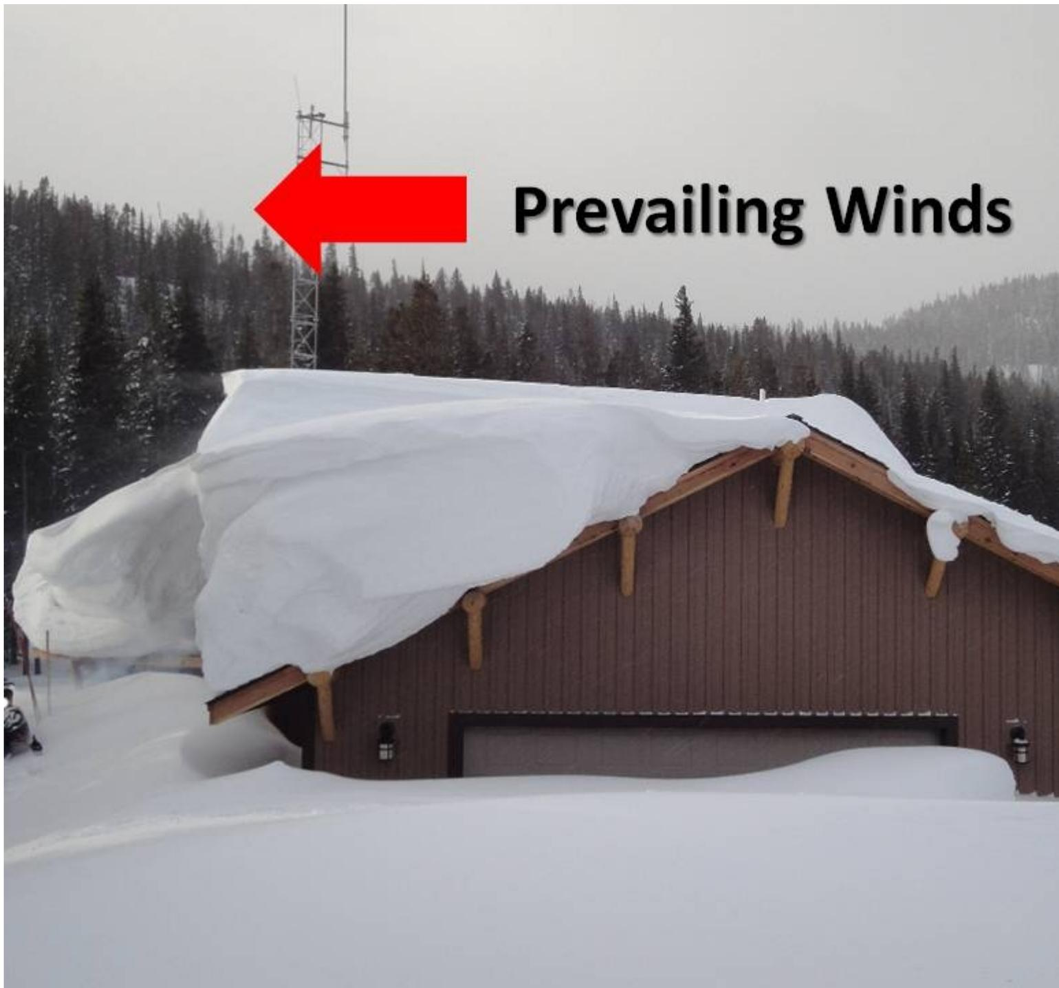
This photo shows the power of the wind to distribute snow. Loading on the lee sides of ridges and roofs can be substantial. Photo: GNFAAC
